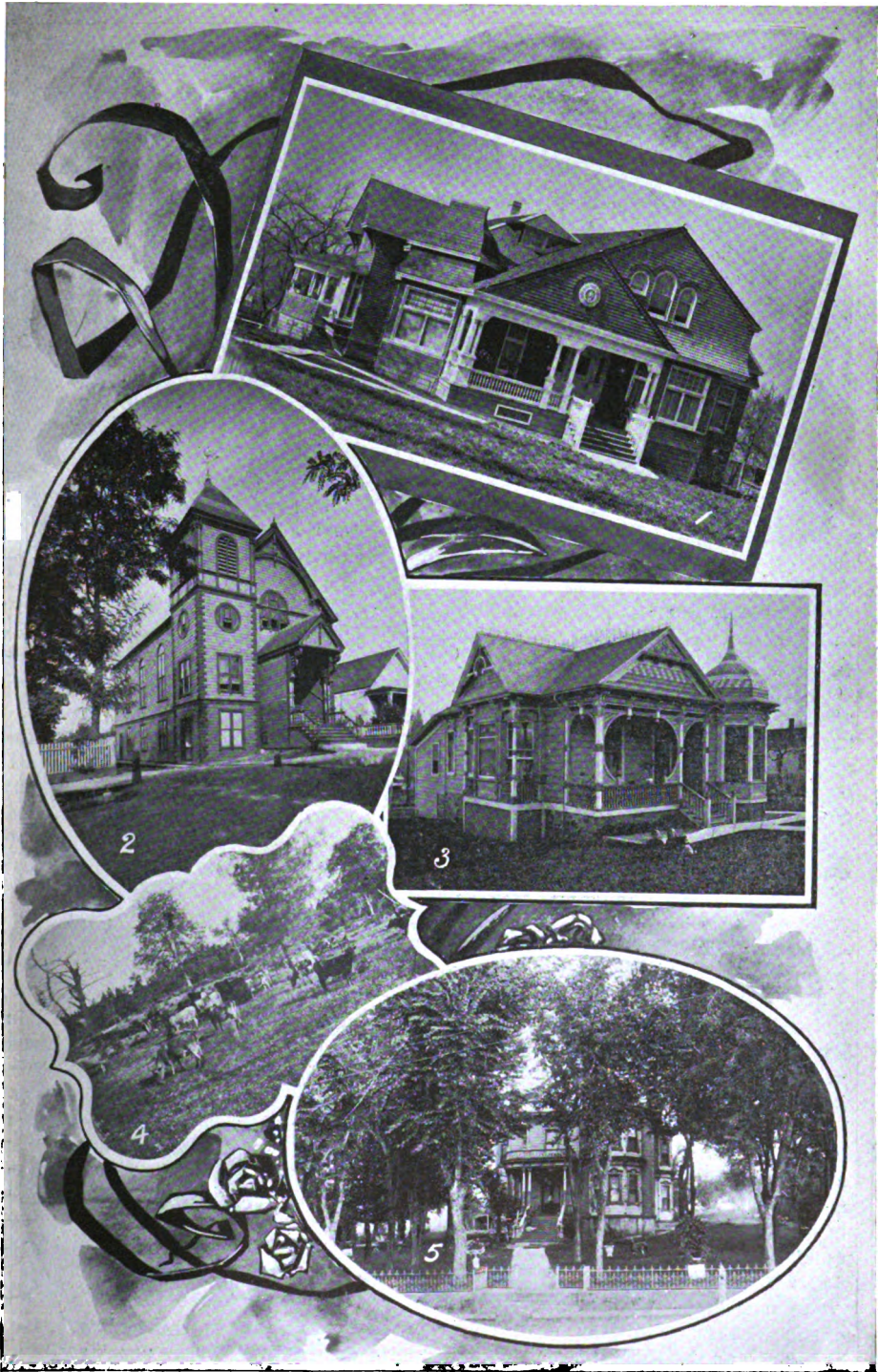
A GROUP FROM NEVADA CITY.—1. A. D. Town's Residence. 2. Methodist Church. 3. Residence of Supervisor W. H. Martin. 4. Sutton's Dairy. 5. Dr. Hunt's Residence.
